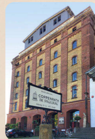
Working behind old walls
